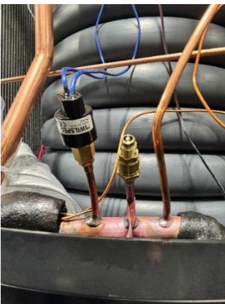
THE L.P. SWITCH HAS BLUE WIRE LEADS
