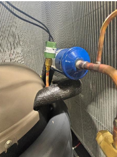
THE HIGH-PRESSURE SWITCH HAS BLACK WIRE LEADS.
